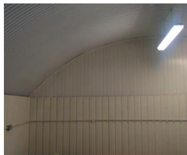
The T & G cladding planks are scribed tight to the arch ceiling sheets – additional capping trim or flashing can be used here if required. Where the planks are not running all the way to the floor they will tuck neatly behind the metal wall sheets.
