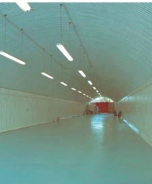
There are 3 lengths of corrugated sheet available to help achieve the optimum material yield; 2.44m, 3.05m and 3.66m. Allowing one corrugation for sheet side-laps, the sheets will have a cover width of 1050mm with respect to the depth of the arch.
